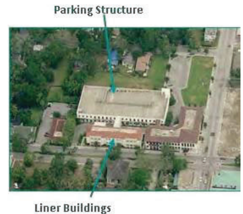
Figure 18. Detached Liner Building
