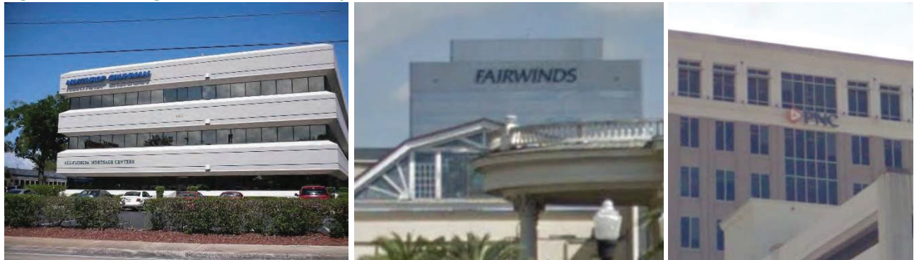
Figure 49. Wall Sign above Second Story
