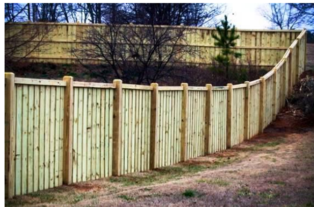
Figure 5.5.8.A: Fence with Finished Side Out
